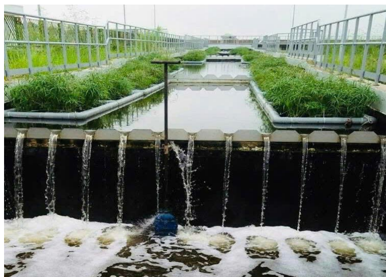
f. Free-floating plant constructed wetland (FFP CW) at Pacific Crystal Textiles Limited, Hai Duong province, Viet Nam.
