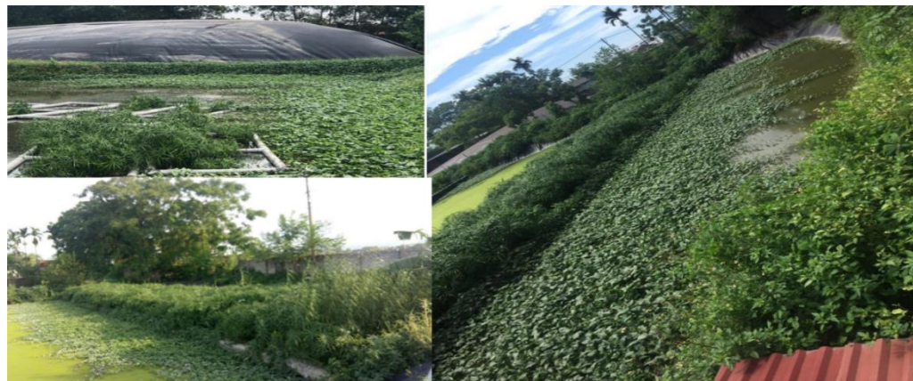
b. Constructed wetlands at a 150 m 3 /day pig farming facility, Tot Dong Commune, Chuong My District, Ha Noi, Viet Nam
