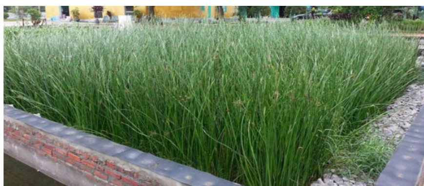
d. Horizontal subsurface flow constructed wetland (HSF CW) system at Quang Ninh Seafood Export Joint Stock Company, Quang Ninh province, Viet Nam.
