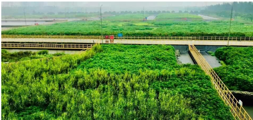
a. Constructed wetlands at Formosa Ha Tinh Steel Corporation, Ha Tinh province, Viet Nam.
